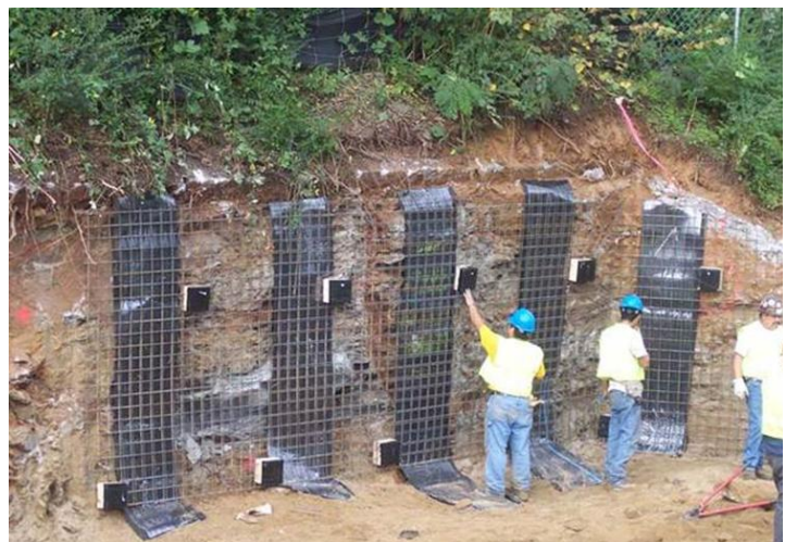
Soil nail walls stabilize hillsides and control erosion
